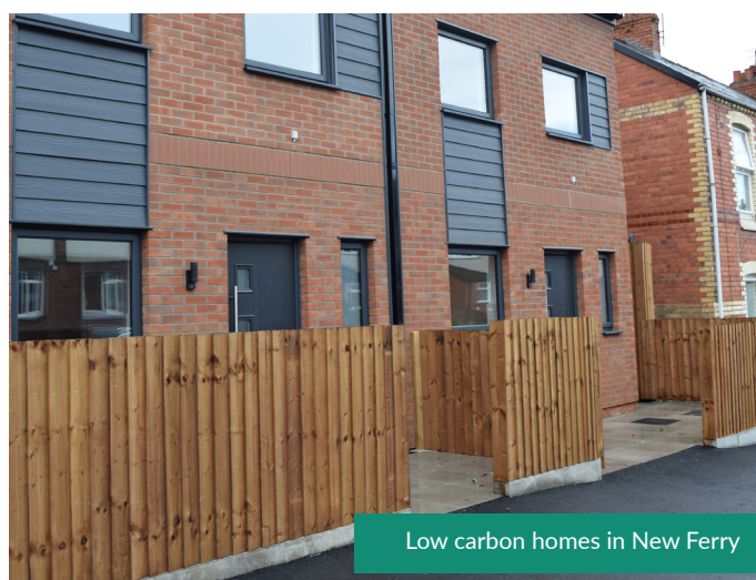
MMC Air Source Heat Pumps at three new properties making them 2050 ready
